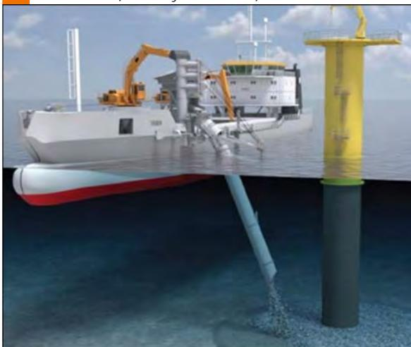
Rock can also be used to backfill a trench that was (for example) created during dredging operations prior to cable installation (Figure 73 and Section 3.7.3). However, it is more commonplace to backfill with the material that was pre-dredged in this situation. The decision to use rock placement as a protection method is usually determined during the permitting phase, typically targets localized areas, and is very rarely used over long distances.
