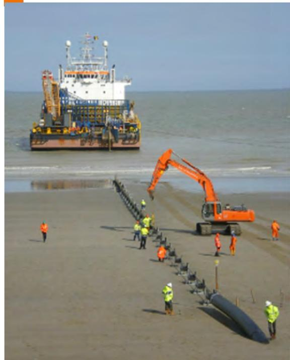
Figure 29. Image Showing Preparations for Pulling the Export Cable into a Plow (Courtesy, VBMS/Boskalis).
