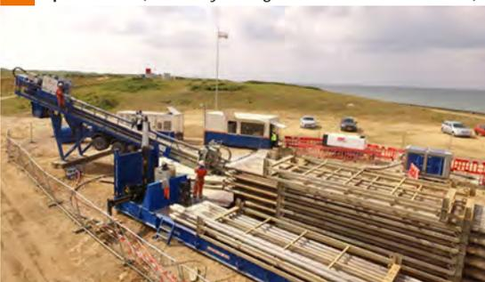
Figure 28. Image Showing Preparations for Pulling the Export Cable into the HDD Duct, with the Offshore End of the Duct Above the Low Water Line (Courtesy, C-Power).
