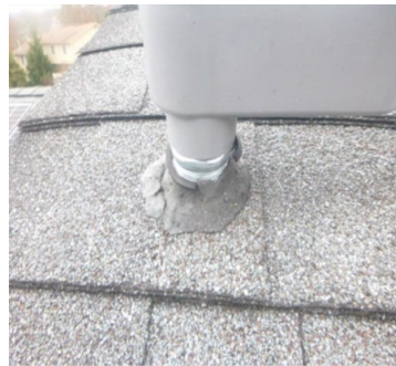
Photo 7: Where not protected from physical damage, equipment grounding conductor must be #6 or larger: NEC 690.46, 250.120(C). Conductors laying on asphalt shingles will become damaged and will not last a PV system's expected 30-year lifespan.
