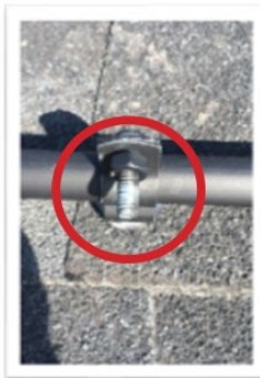
Photo 7: Where not protected from physical damage, equipment grounding conductor must be #6 or larger: NEC 690.46, 250.120(C). Conductors laying on asphalt shingles will become damaged and will not last a PV system's expected 30-year lifespan.
