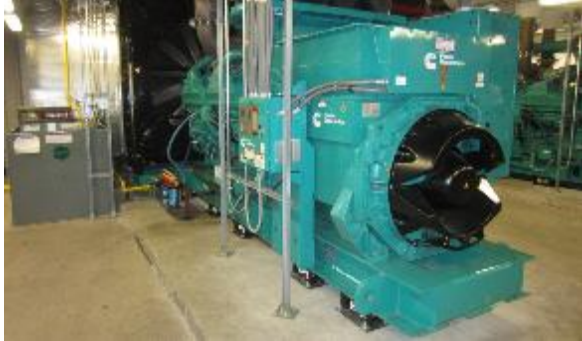
Figure 2.36. MV Generators
