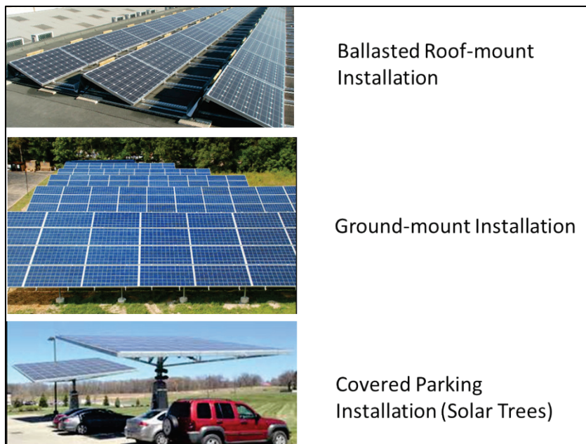
Figure 13 – PV Installation Options.
