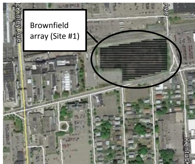
Figure 16: Brownfield PV array
