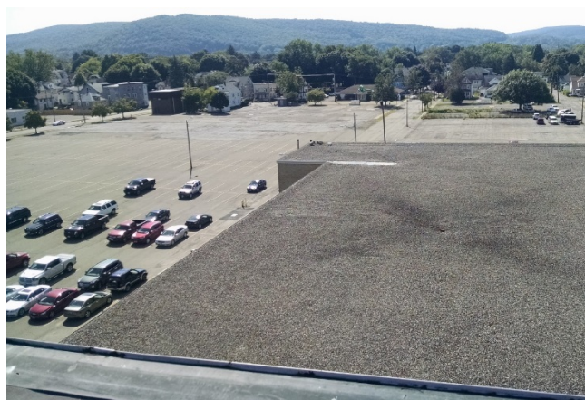
Figure 19: Adams Ave Carport site seen from Bldg 40
