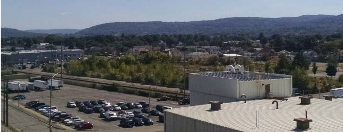
Figure 17: Brownfield as seen from Building 47 rooftop.
