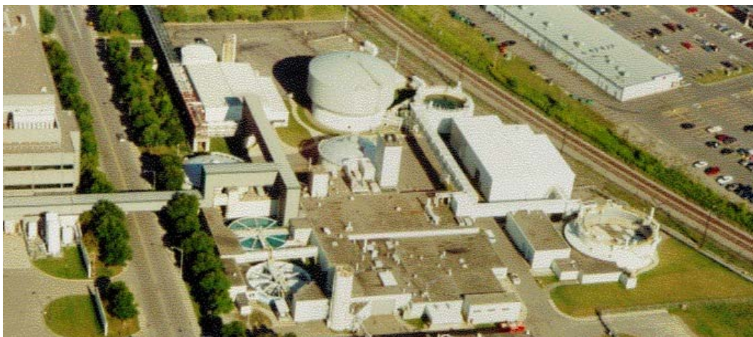
Figure 22: Huron Campus Wastewater Treatment Plant
