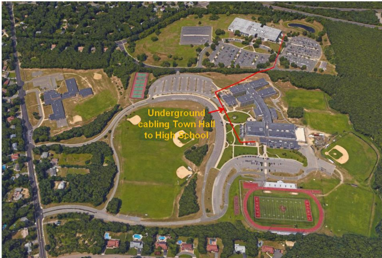
Photo 2-6. Underground Cabling Between Town Hall and High School
