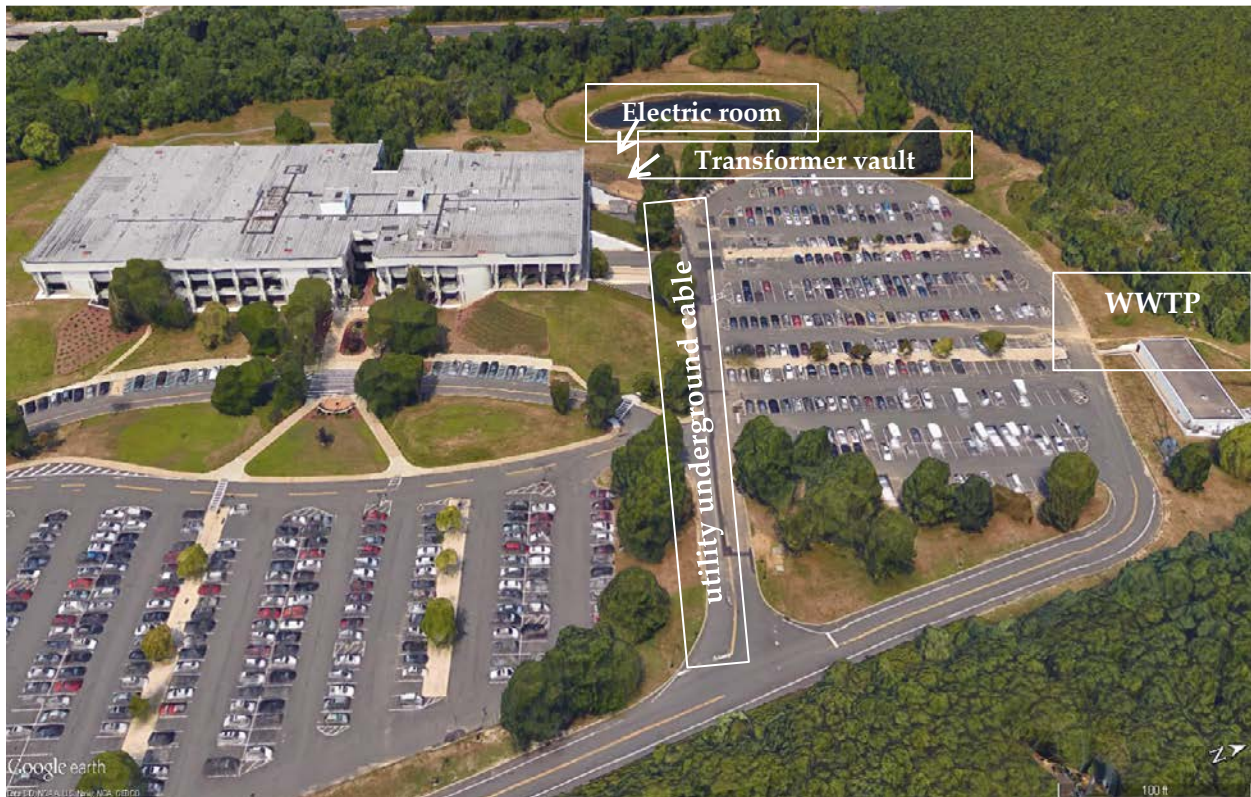
Photo 2-3. Brookhaven Town Hall
