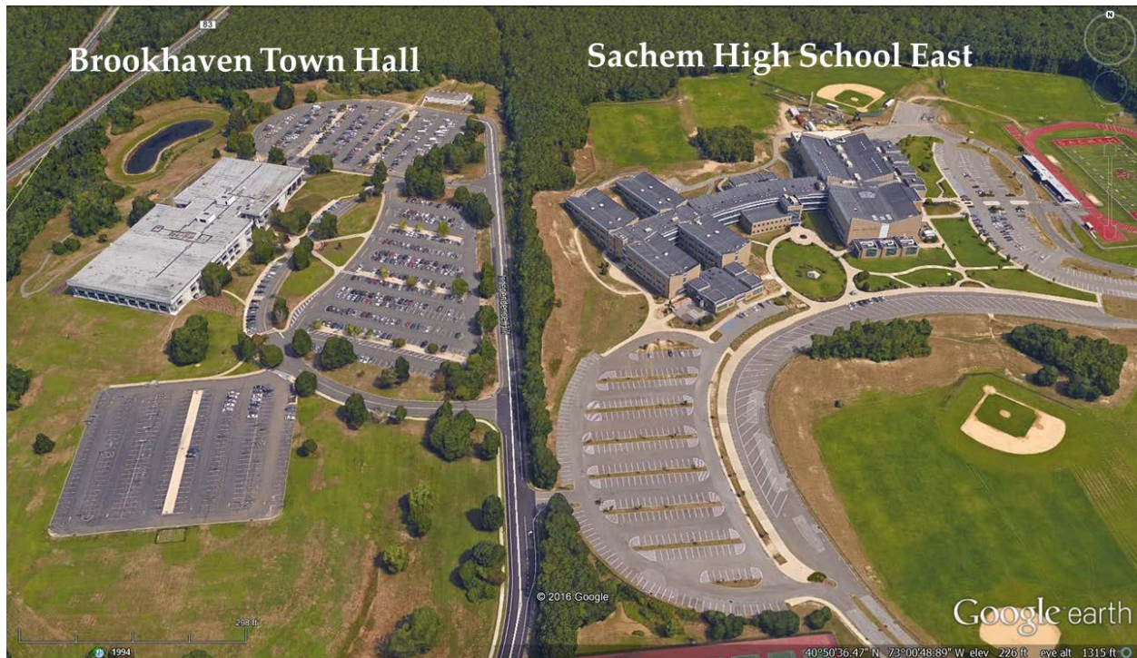
Photo 2-2. Brookhaven Microgrid Site Overview
