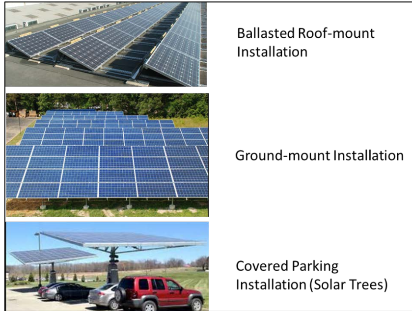
Figure 14 – PV Installation Options.
