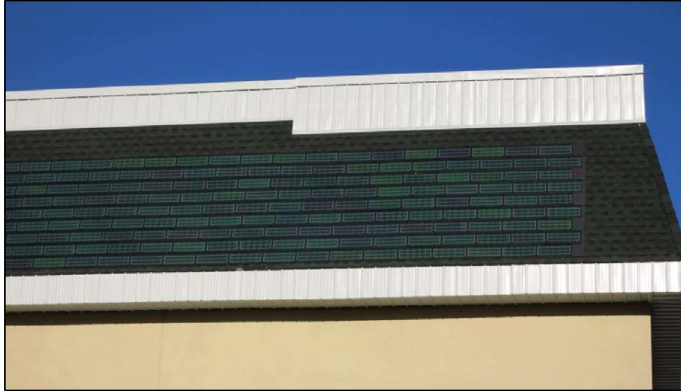
Figure 18. 8kW PV array at Mamaroneck Self Storage
