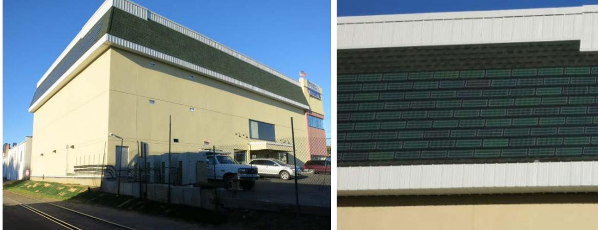
Figure 13. (left) General exterior (right) Solar shingles
