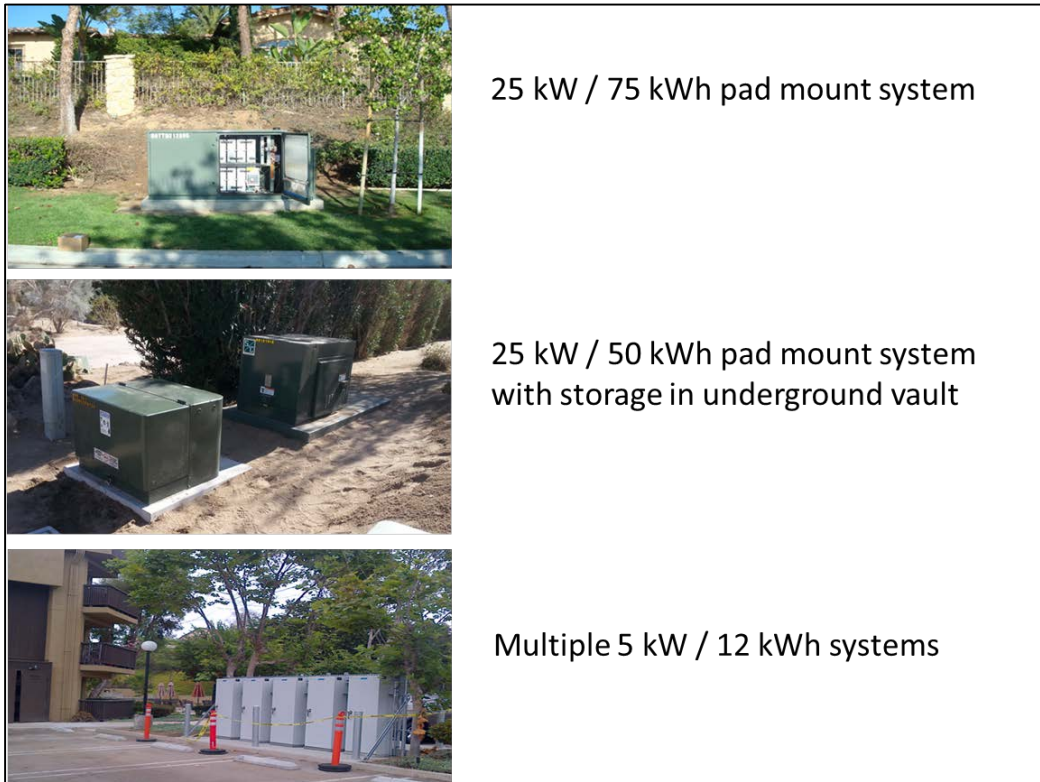
Figure 17 – Example ESS Installations
