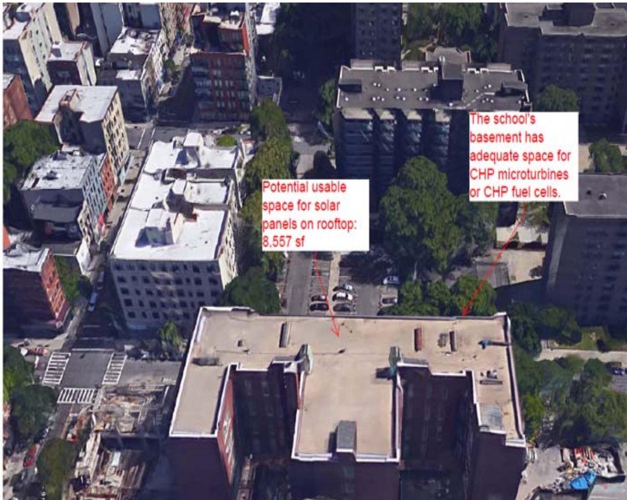
Figure T1-16 East Village Community School, Building E
