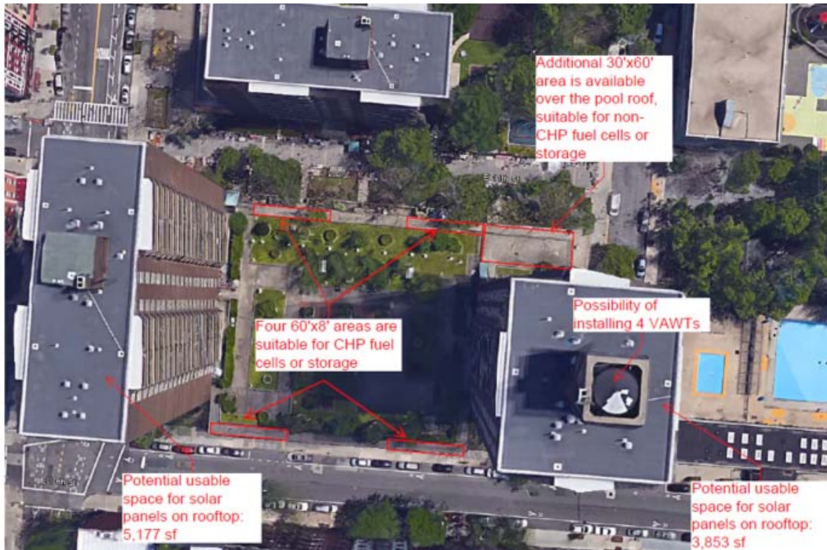
T1-17 Village East Towers (South) – Building G and H
