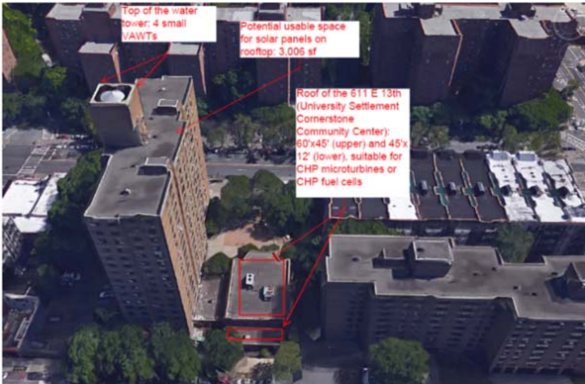
T1-14 Campos Plaza II West Side – Building A
