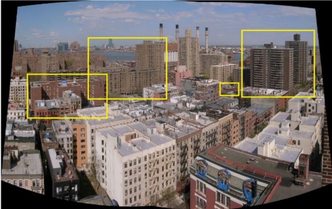
Figure T1-1: Looking north east across the Two Bridges/Beyond the Grid Community Microgrid Project Area, with participating sites outlined.
