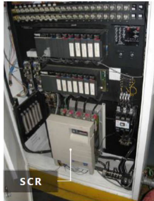
Figure 2b: Elevator control with solid state rectifier—the controller panel has been opened to show the interior. Silicon-controlled rectifiers (SCRs) are a common form of solid state rectifier. The SCR serves the same function as the older-style rectifier (Figure 2a).
