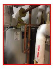
*Incorrect:* Improper and/or incomplete pipe insulation was seen on site.
