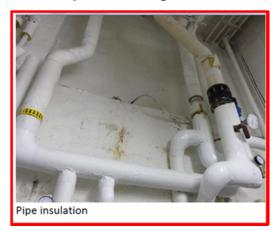
*Incorrect:* This photo shows the location of piping and correctly installed pipe insulation, but an additional photo showing pipe insulation thickness is required.
