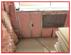
*Incorrect:* This photo shows poorly installed interior batt insulation, which is slumping and protruding between the studs. This does not meet RESNET standards or program requirements.
