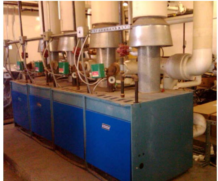
Fig. 2 Cast Iron Sectional Boilers
