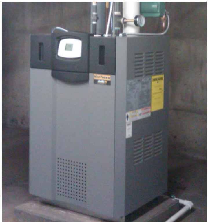
Fig. 3 New condensing boiler
