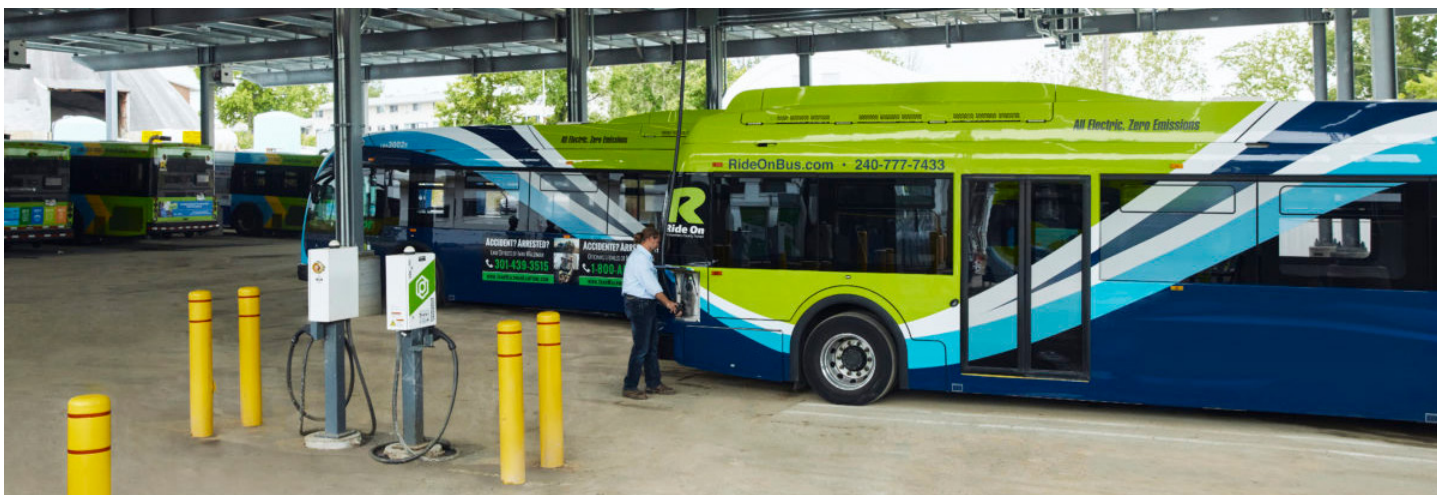
This bus depot in Maryland shows pedestal mounted and overhead dispenser chargers. Overhead dispensers can be used when a roof structure is present to minimize the chargers' footprint. Source: Mobility House
