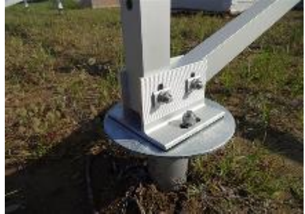
Mounting on top of Ground screw
