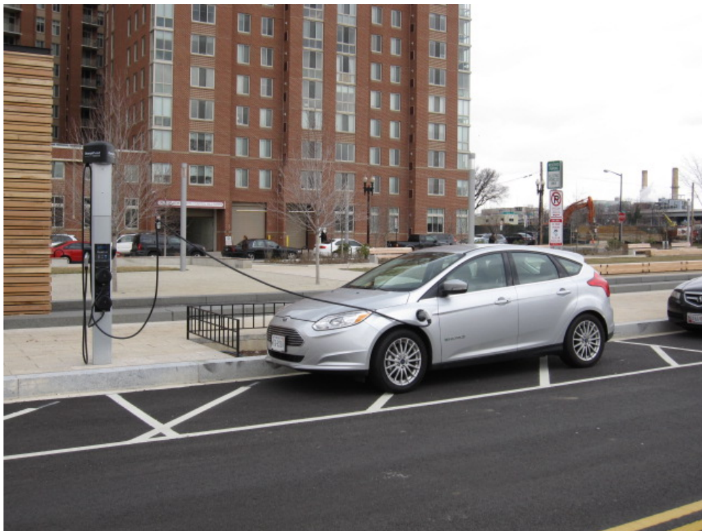
Figure 17. Charging station at Canal Park
