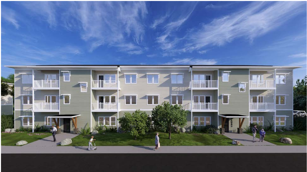
EcoFlats Typical 12-Unit Building | Black Mountain Architecture
