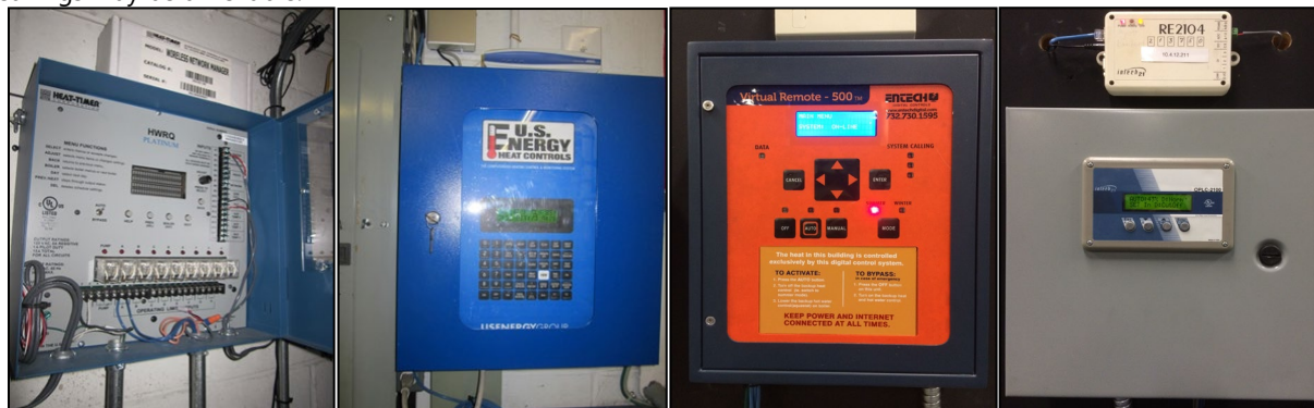
Figure 1: Central computers of Energy Management Systems installed in the field and manufactured (from left to right) by Heat-Timer, U.S. Energy, EnTech, and Intech 21. Photo credits: Far left and left by Taitem Engineering; right and far right by the Association for Energy Affordability
