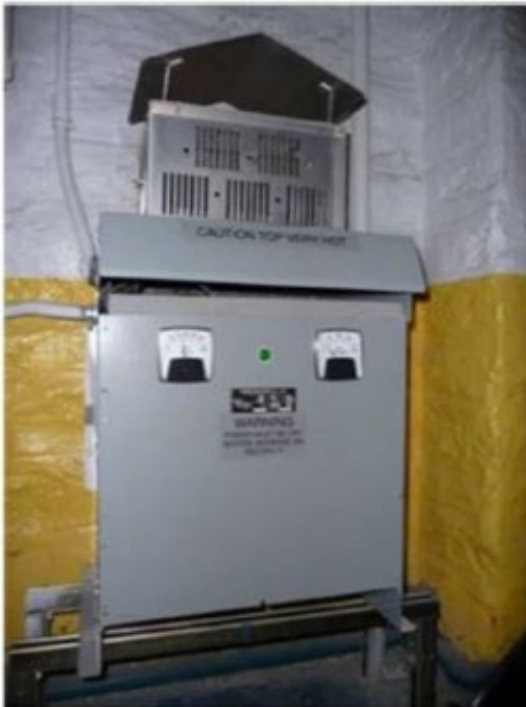
Figure 2a: Rectifier, not solid state. This old-style rectifier is roughly the size of an under-counter refrigerator
