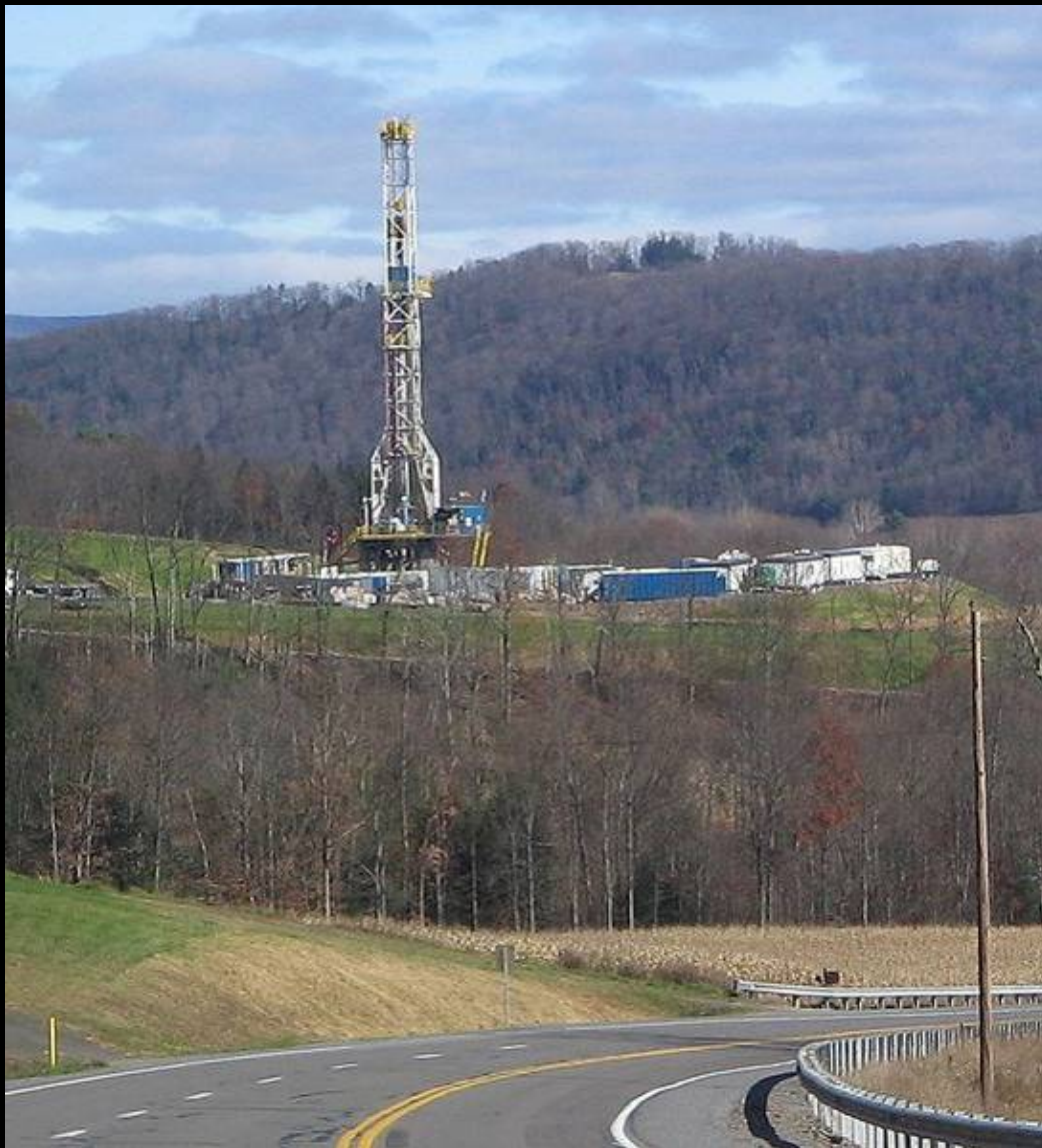
Drilling Rig- This is only present for the drilling of the well(s) and is then moved on to the next well
