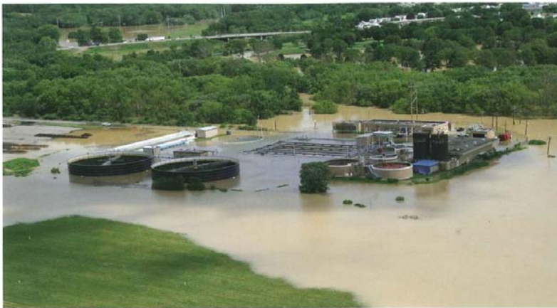
The flood of 2006 overwhelmed the Endicott Sewage Treatment Plant.
