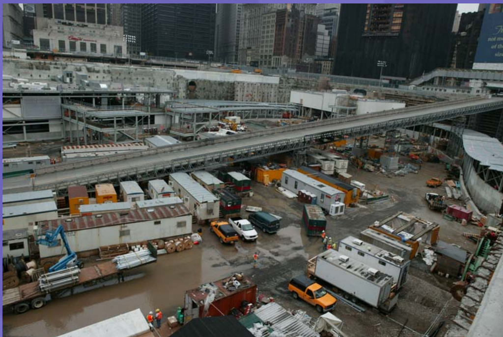
Trucks Delivering Material to WTC Site
