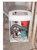
Low NO x (Blue Flame) Burner
