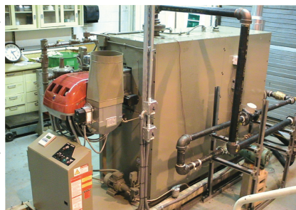
A B100-fired boiler in a Brookhaven National Laboratory testing facility
