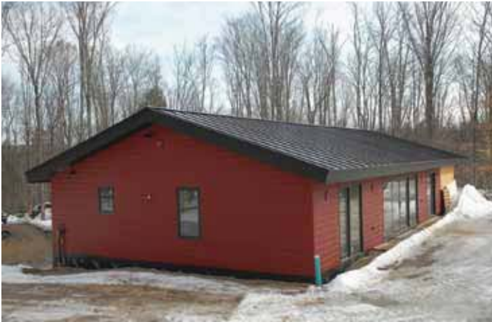
Single family home constructed in Tupper Lake, New York, contains ICF foundation and walls with 12" SIP roof, heating provided by small boiler with radiant floor heat. Whole house ventilation serves the IAQ, occupant energy usage after two years is 65% below average consumption.
