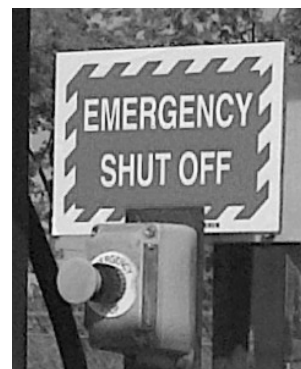
Figure 13. Emergency shut-off buttons for compressed natural gas maintenance facilities and fueling infrastructure
