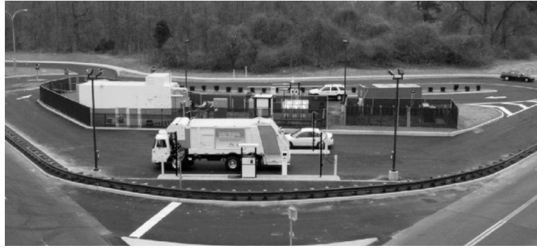
Figure 26. Hauppauge fast-fill compressed natural gas station
