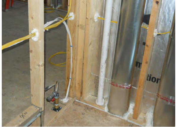
Plumbing, electrical and HVAC penetrations between floors.
