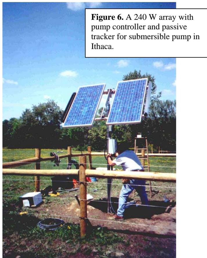
**Figure 6.** A 240 W array with pump controller and passive tracker for submersible pump in Ithaca.
