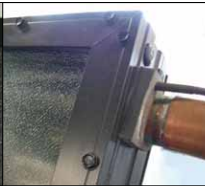
Figure 1-23 – Sensor installed in collector dry well. The well is partially visible behind the glazing.
