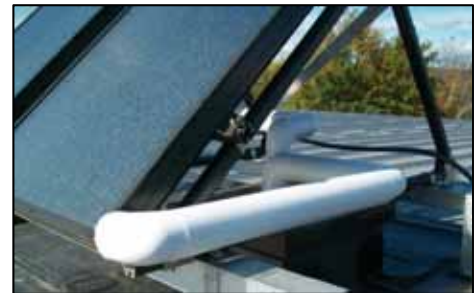
Figure 1-37 – PVC cladding over exterior insulation
