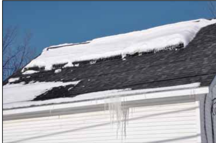
Figure 1-6 - Evacuated tube collectors flush-mounted on a roof with an 8:12 slope (photo courtesy of Kennebec Valley Community College)
