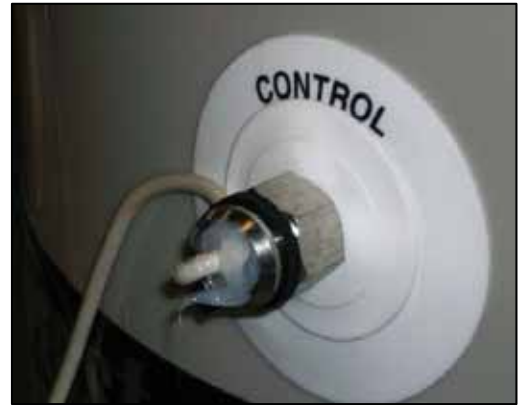
Figure 3-5 – Properly installed sensor in immersion well. Care must be taken to ensure bend in sensor wire is at an appropriate radius.
