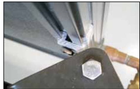
Figure 1-26 – Set-screw style collector attachment
