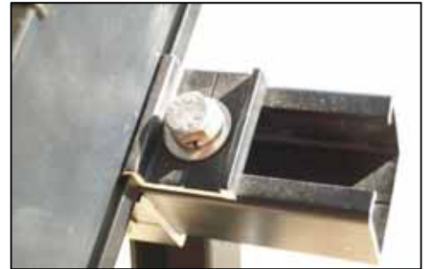
Figure 1-25 – Clamp style collector attachment
