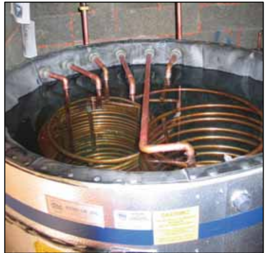
Figure 3-4 – Interior view of unpressurized tank (image courtesy of Liquid Solar Systems).
