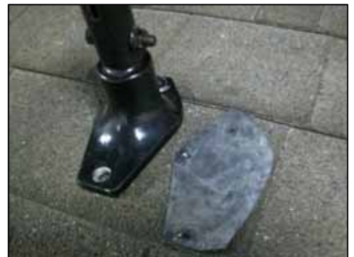
Figure 1-36 – Custom EPDM gasket for mounting foot. Sealant should be applied between gasket and roof and gasket and foot before installing the lag screws.
