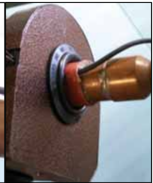
Figure 1-24 – Sensor installed between header and heat shield (sensor wire must be secured to piping and have a high-temperature coating)
