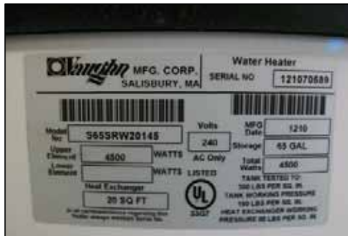
Figure 3-2 – Manufacturer's label with information regarding the model and storage capacity
