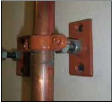
Figure 2-1 – Split ring, threaded rod, and plate
