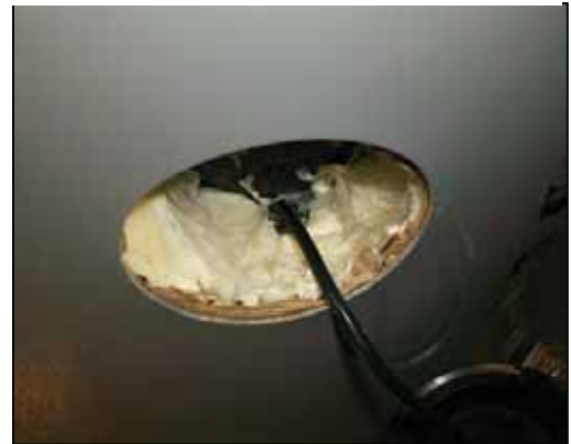
Figure 3-6 – Sensor placed between insulation and vessel wall. This area should be insulated before replacing plastic cap to limit heat loss and increase accuracy of sensor location.
