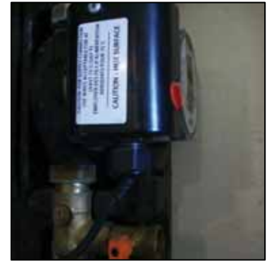
Figure 4-1 – Strain relief clamp used at circulator junction box to protect the integrity of the corded connection.
