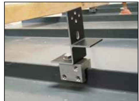
Figure 1-31 – Standing seam clamp attached to collector bracket
