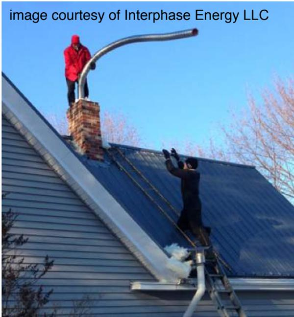
stainless steel rigid liner pipe joined with stainless steel pop rivets
