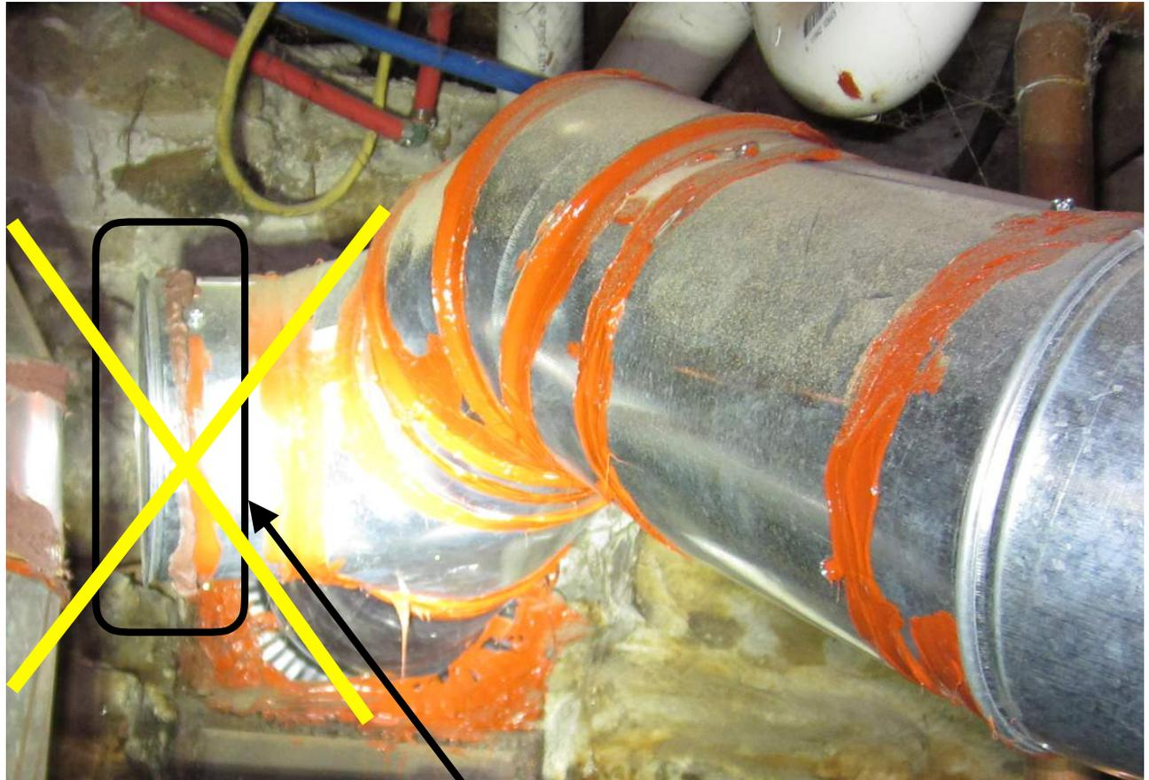
Standard barometric damper was removed and opening sealed because of ash and flue gas leakage.
