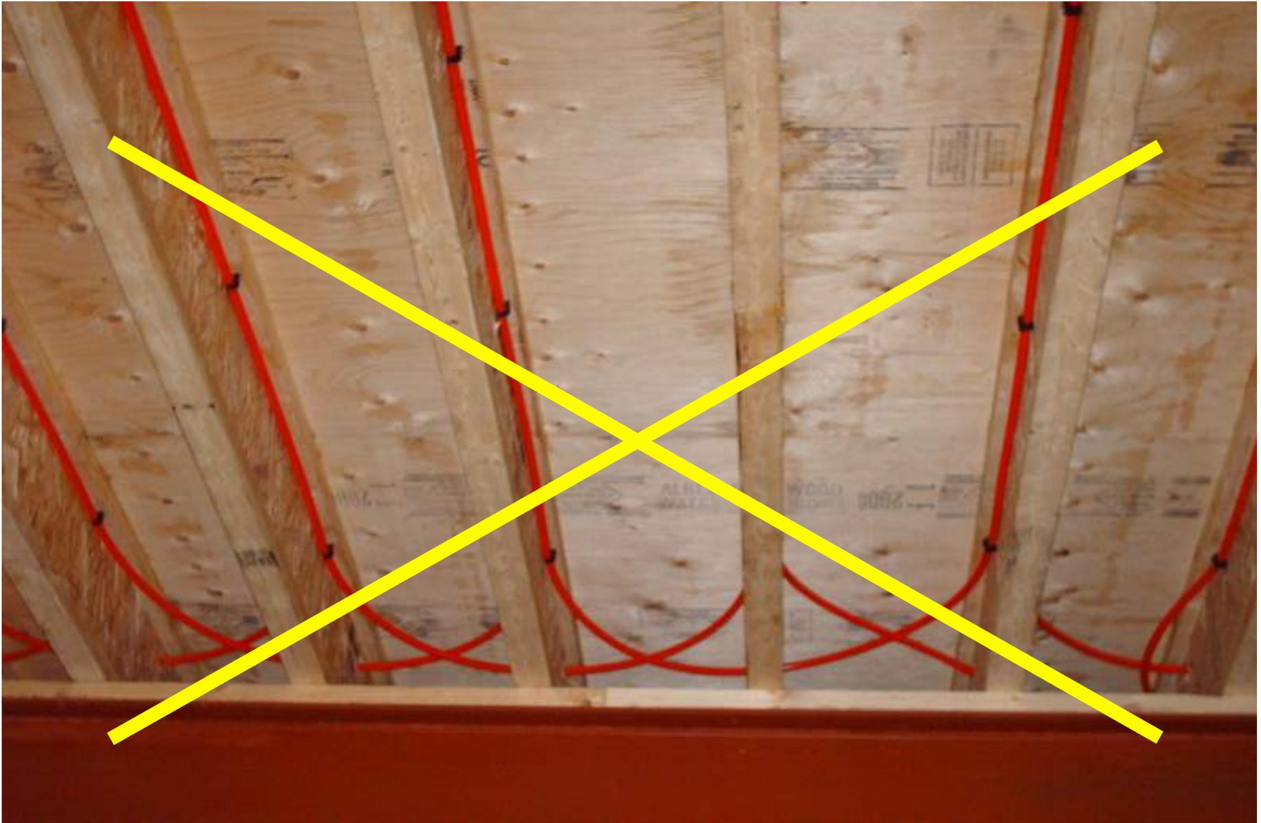
Heat transfer between the water and the upper floor surface is severely restricted!
