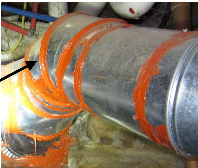
RTV silicone. Will eventually separate from galvanized pipe
