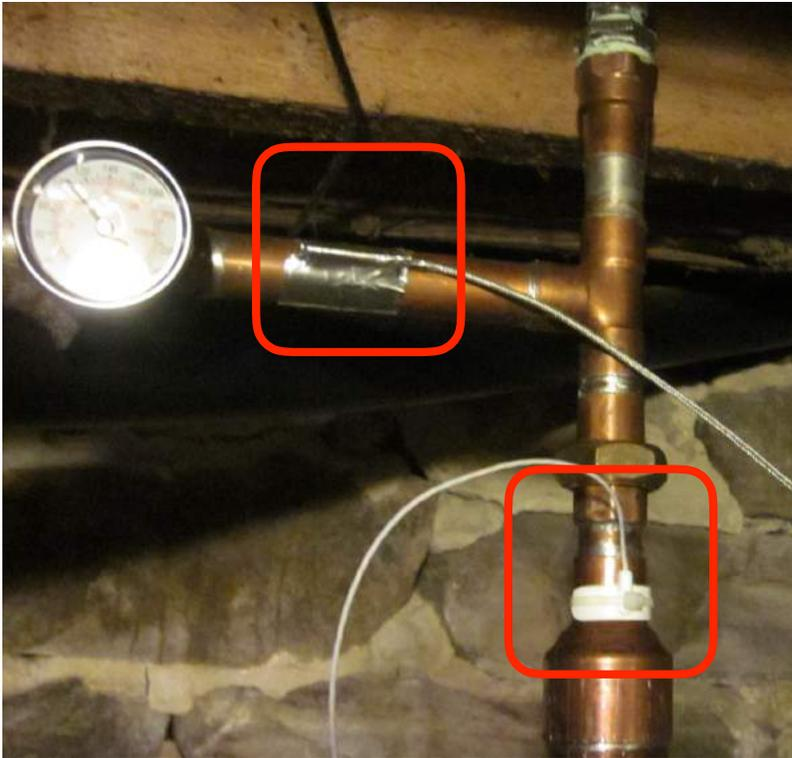
non-insulated surfaced mounted temperature sensors
