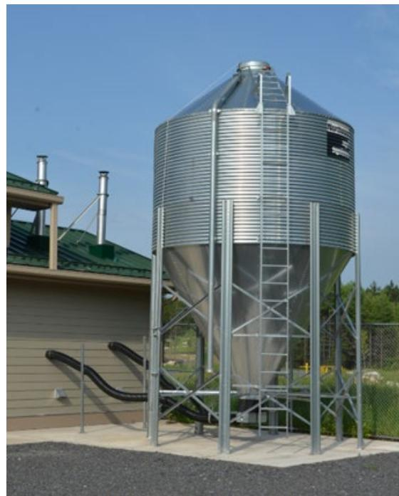
**Figure 3-9. Polyethylene pellet storage silo**
