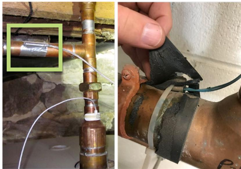
The temperature sensor seen inside the green box of Figure 7-35 is taped to the copper tubing. The intended purpose was to measure water temperature in the upper portion of a thermal storage tank—the top of which is seen just below the piping. Instead, this sensor is measuring a temperature somewhere between that of the tube surface and the surrounding air. The pellet boiler in this system was fired based on the temperature of this sensor. Boiler operation was not as expected.
