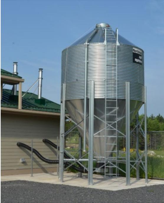
**Figure 3-9. Polyethylene pellet storage silo**
