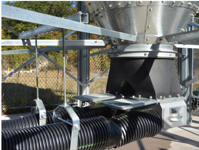
All tubing used for pneumatic pellet transfer should have a ground wire that's attached to the pellet boiler chassis, which itself is connected to an electrical ground. Electrical grounding drains away static electrical charge that could otherwise build up from dust moving along with the high-speed air through the pellet transfer tubing. See the pellet boiler's installation instructions for details on properly grounding the pellet transfer tubing.
