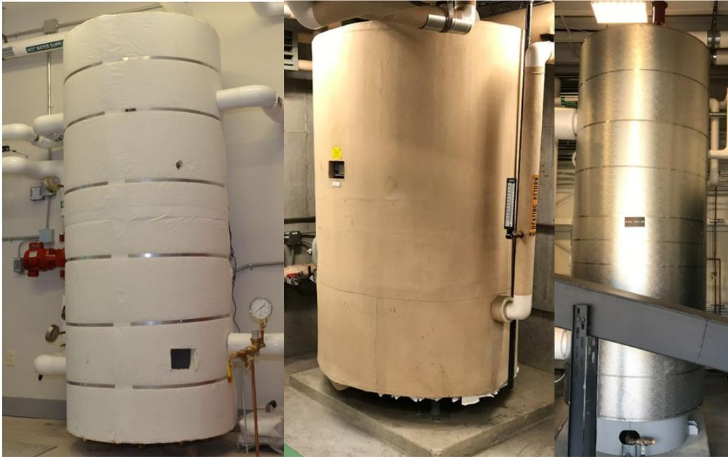
All three tanks have site-installed insulation. The tank on the left and in the center have reinforced fabric jackets to protect the insulation. The tank on the far right uses an aluminum sheet metal jacket to protect the insulation.
