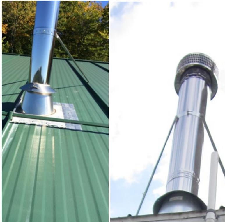
All braces should be secured directly to building structural elements (rafters, trusses, etc.) using stainless-steel hardware and grommets or sealants to waterproof all roof penetrations. Another possibility is to install a snow splitter upslope from the chimney as seen in Figure 4-7.
