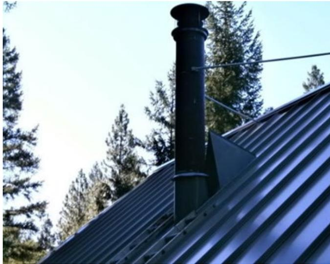
Snow splitters are designed to deflect sliding snow around the chimney and its flashing. Splitters should be made of materials such as aluminum or stainless steel in thickness that can handle substantial force without bending. Snow splitters should also be anchored to building framing using multiple stainless-steel fasteners.
