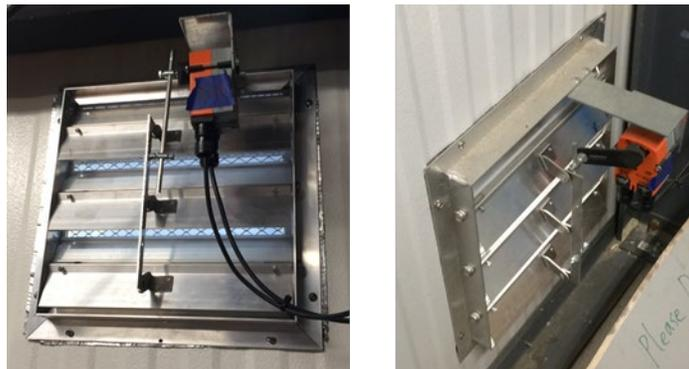
If motorized dampers are used, codes require that their actuators are equipped with “end switches” that close only when the damper is fully open. These end switches should be wired in series. The series-connected end switches must then be wired into the boiler’s control system so that the boiler cannot fire if the dampers fail to open or fail to remain open.
