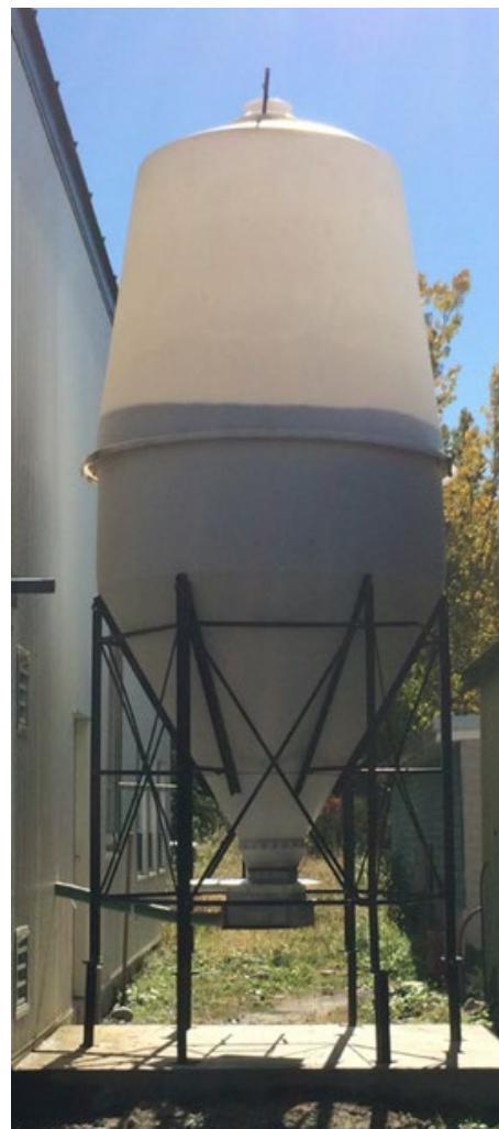
It's also possible to measure the pellet contents of a storage silo by suspending the silo on load cells, which send electrically encoded signals based on the weight they support. Figure 3-21 shows an example of a custom-built pellet silo suspended on four load cells.
