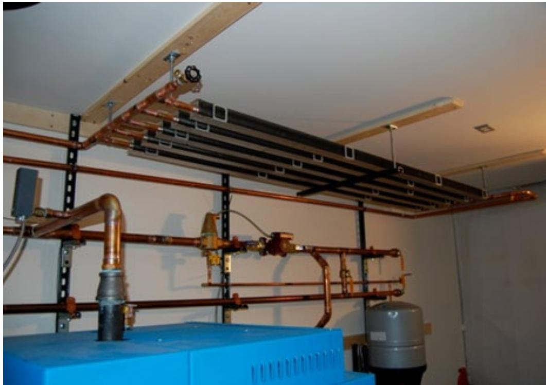
The finned-tube array is installed above the boiler and connected to the boiler's supply and return piping. It should have a slight downward slope in the direction of flow to encourage air bubbles to rise to a high-point vent or bleeder valve.
