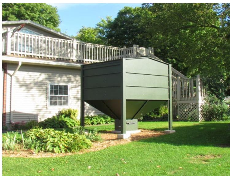
It's also possible to construct an exterior pellet storage bin from common building materials. An example is shown in Figure 3-7
