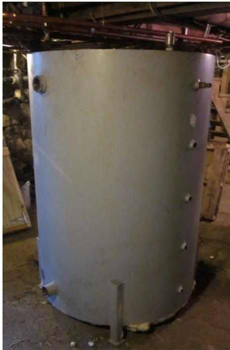
Because of the water volume they add to the system, the system's expansion tank must be significantly larger than for an equivalent system without thermal storage. A starting estimate for the size of the expansion tank is 10% of the volume of the thermal storage tank. Floor mounted expansion tanks are typically used due to the required size and weight.
