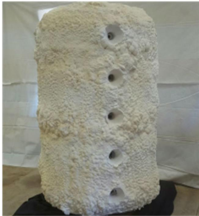
The foam insulation has been held back at all piping connection points. This allows easier attachment of the piping as well as a “receptacle” to support the end of piping insulation. Any unused tappings on the tank can be plugged and then covered with insulation.
