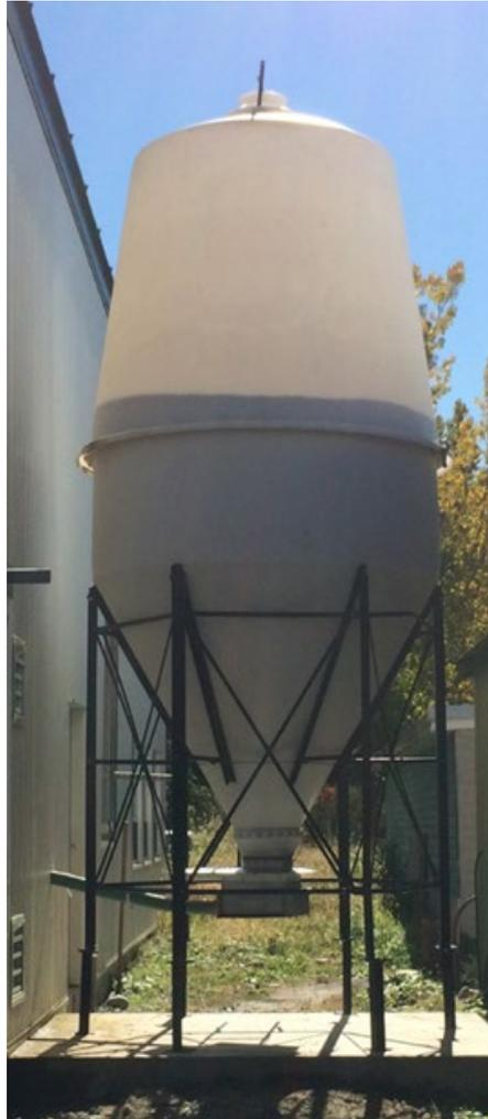
It's also possible to measure the pellet contents of a storage silo by suspending the silo on load cells, which send electrically encoded signals based on the weight they support. Figure 3-21 shows an example of a custom-built pellet silo suspended on four load cells.
