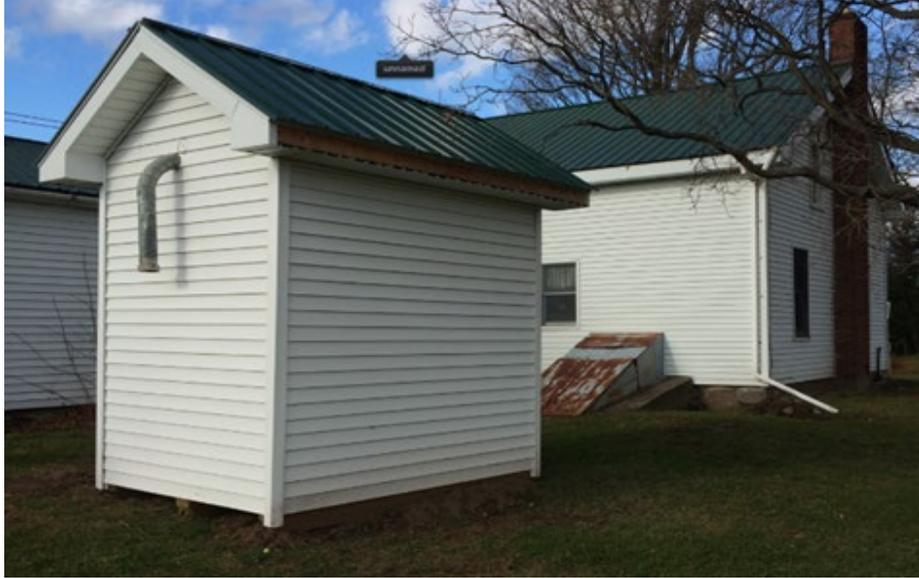
The pellet storage building in Figure 3-7 has interior sloping plywood surfaces that form a hopper to channel pellets into a steel receiver at the base. The pellets are pulled from this receiver into the building through underground tubing routed through PVC protective sleeving.
