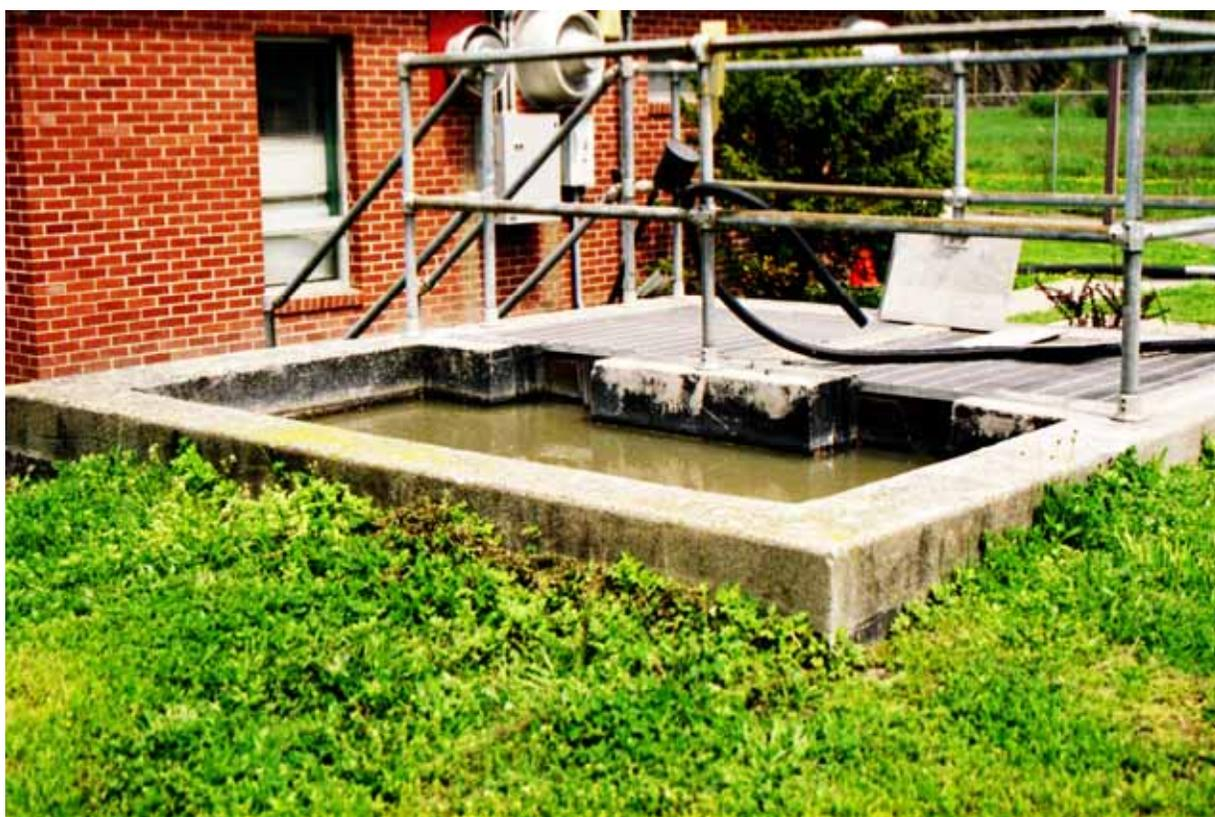
Figure 5-2. V-notch Weir Plates in Flow Splitter Box
