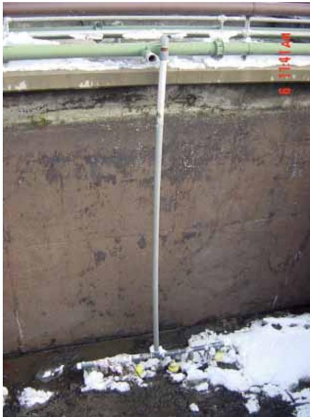
Figure 5-5. Modified Influent Piping for Selector-Contact-Stabilization Demonstration
