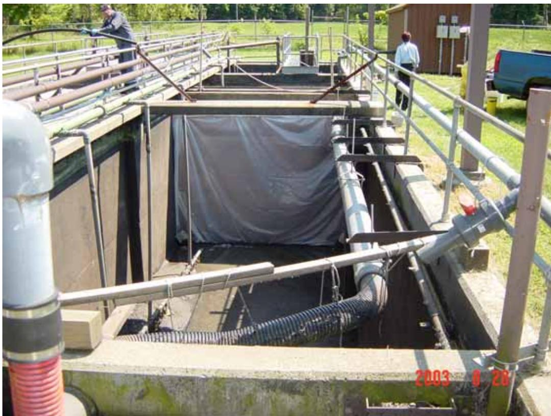
Figure 6-4. Installing Fiberglass Sheeting on the Baffle Wall Face
