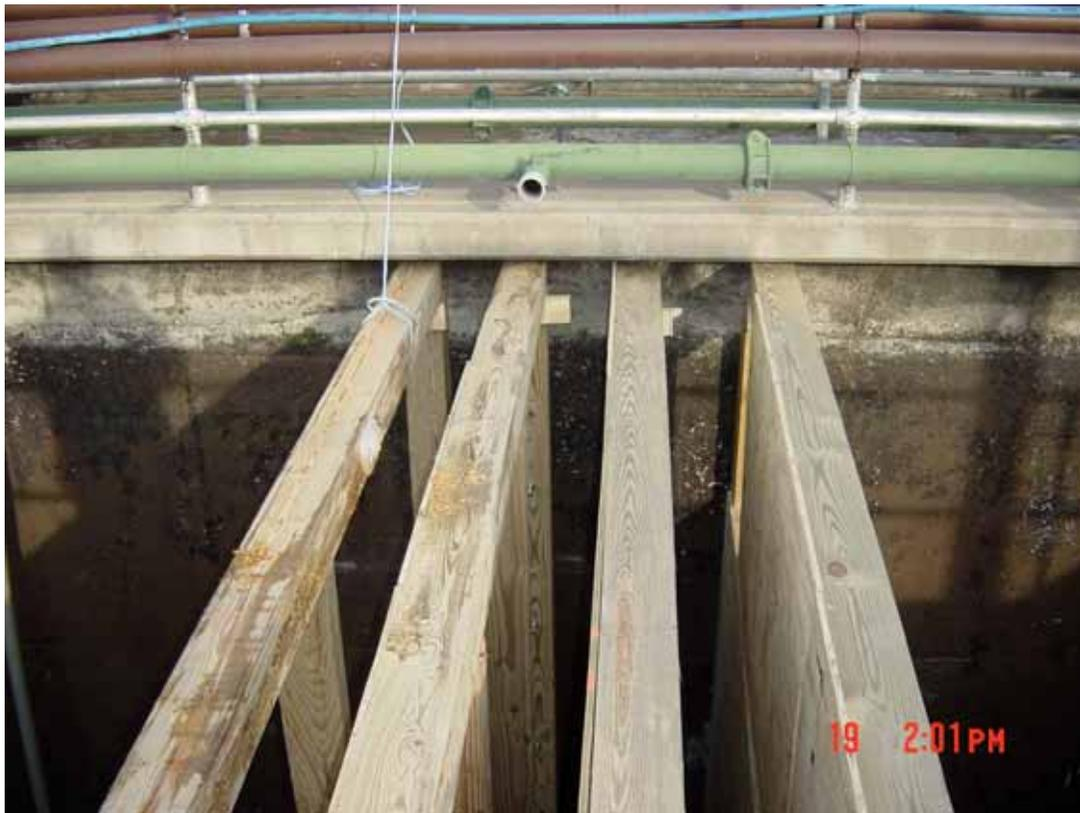
Figure 5-4. Aeration Header in SCS Modified Tank
