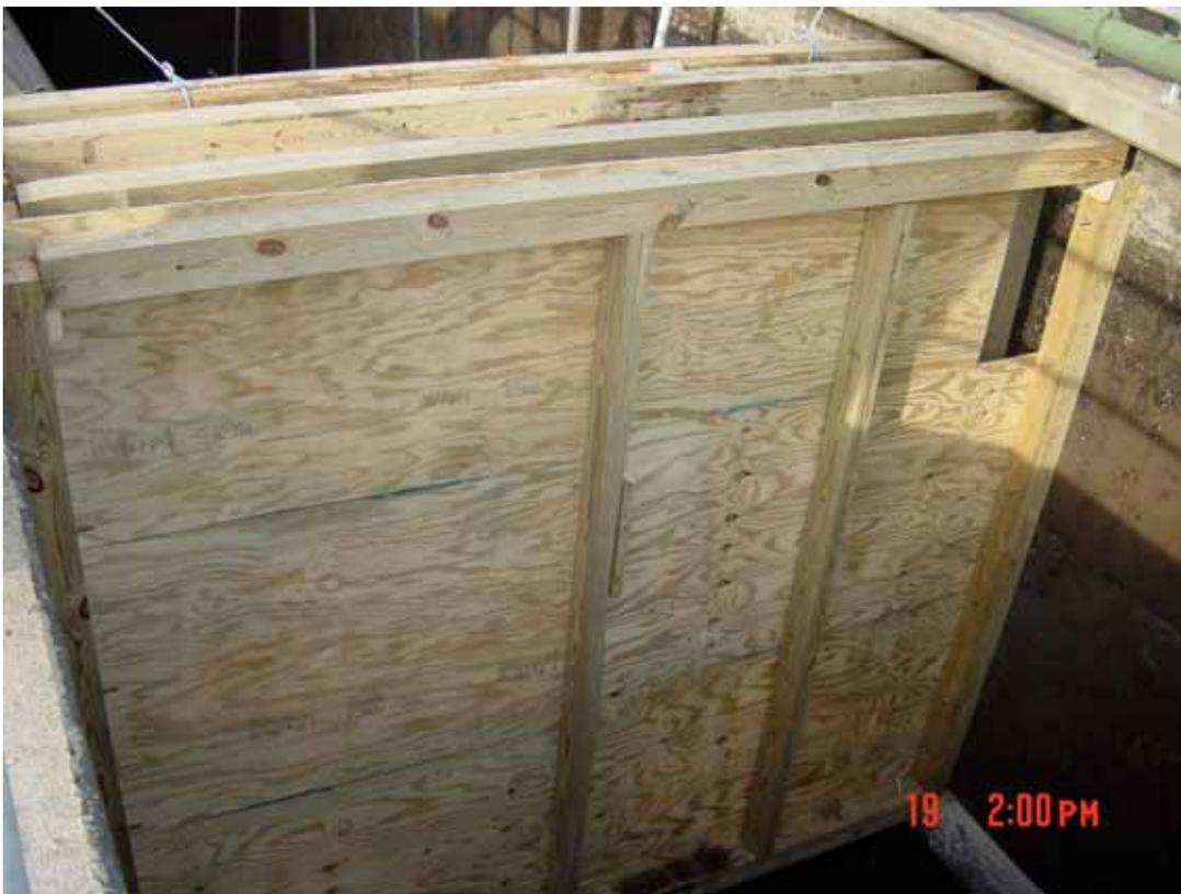
above a concrete fillet that ran along the bottom edge of the sides of the aeration basin, which left a large gap underneath each baffle wall (see Figure 6-2). Short-circuiting between the different zones was occurring through these gaps.
