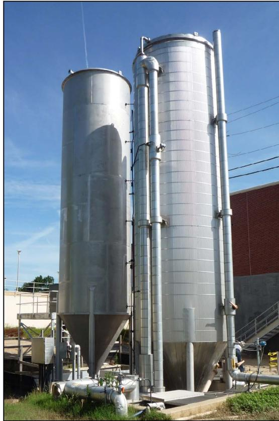
Figure 3-2. SCWRF Plug Flow Reactors during Construction.
