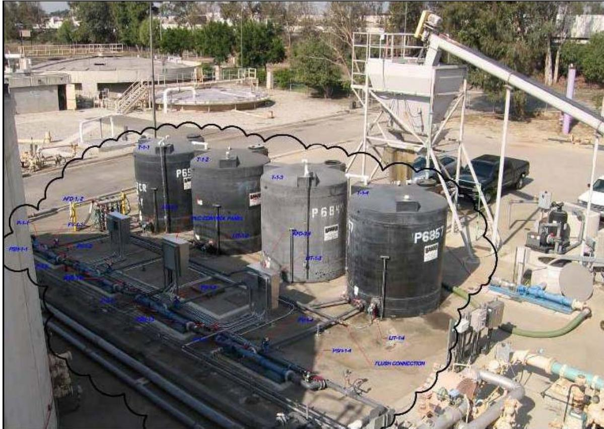
Figure 3-5. Food Waste Receiving Tanks, Test Digester (Digester 4), and Piping Modifications for Pilot Co-digestion Project In IEUA RP-1.
