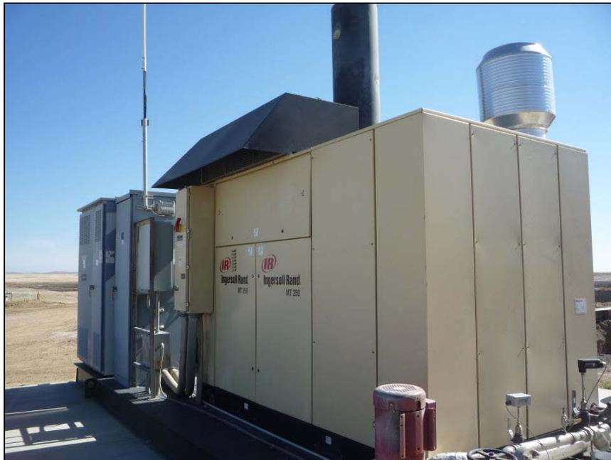
**Figure 3-14 Ingersoll-Rand – MT 250 Microturbine at the Lancaster WRP.**
