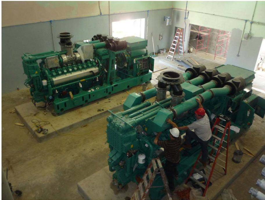
**Figure 3-3. SCWRF Engine-Generators during Installation.**
