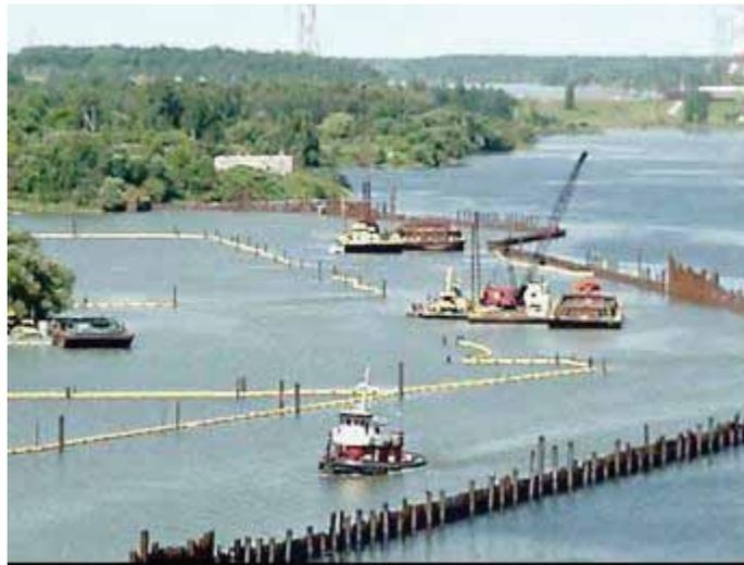
**Figure 2-5. Fixed Sheet Piles**
