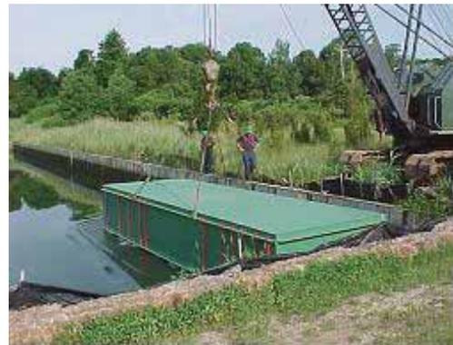
**Figure 3-3. Sectional Barge Shore-side Deployment**
