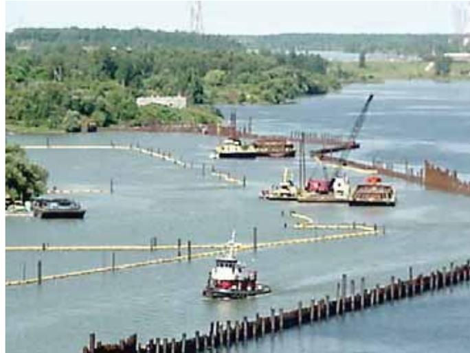
**Figure 2-5. Fixed Sheet Piles**
