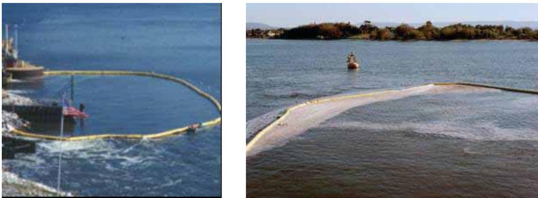
**Figure 2-4. Silt Curtains**
