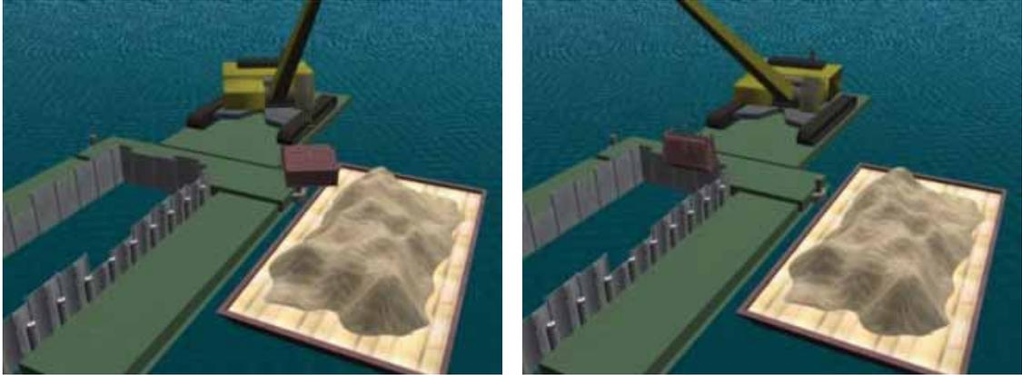
**Figure 5-1. Capping Operation**
