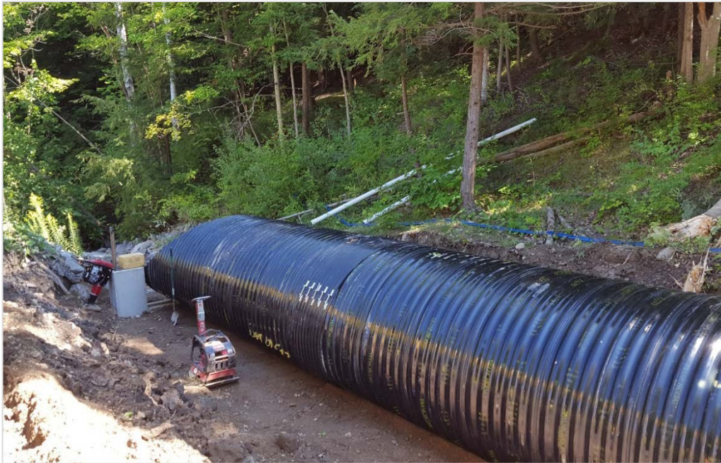
Figure 4-2. Completed CMP installation and Restoration
