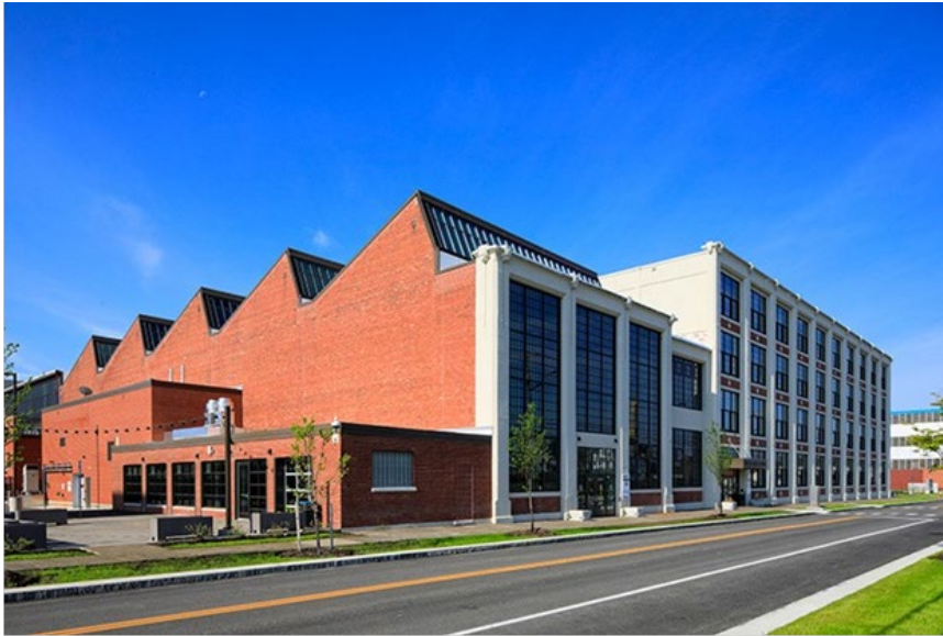
Figure 1. Northland Workforce Training Center, Exterior View
