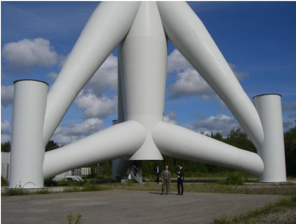
The tripod is installed by driving three piles into the each of the three legs of the prefabricated substructure. It does not require as heavy, or as specialized, pile driving equipment as a monopile. The use of suction buckets rather than piles is a possible alternative to avoid shallow bedrock (Jiang 2021).
