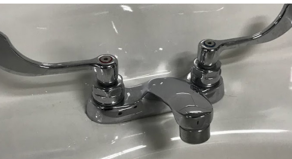
Farmingdale State College (SUNY) installed over 250 low flow aerators on faucets across campus. Credit: Farmingdale State College (SUNY)
