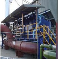
Most Environmental Agencies require all air emissions to be heated to 850°C for more than 2 seconds, typically requiring high energy consumption.
