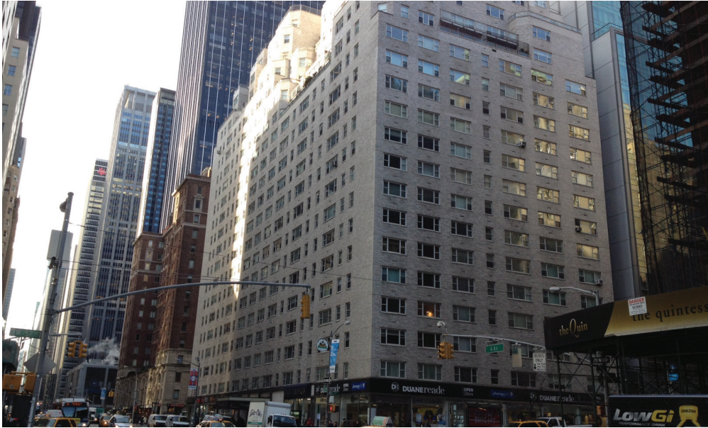
Carnegie House, Manhattan, NY. Photo credit: NYSERDA
