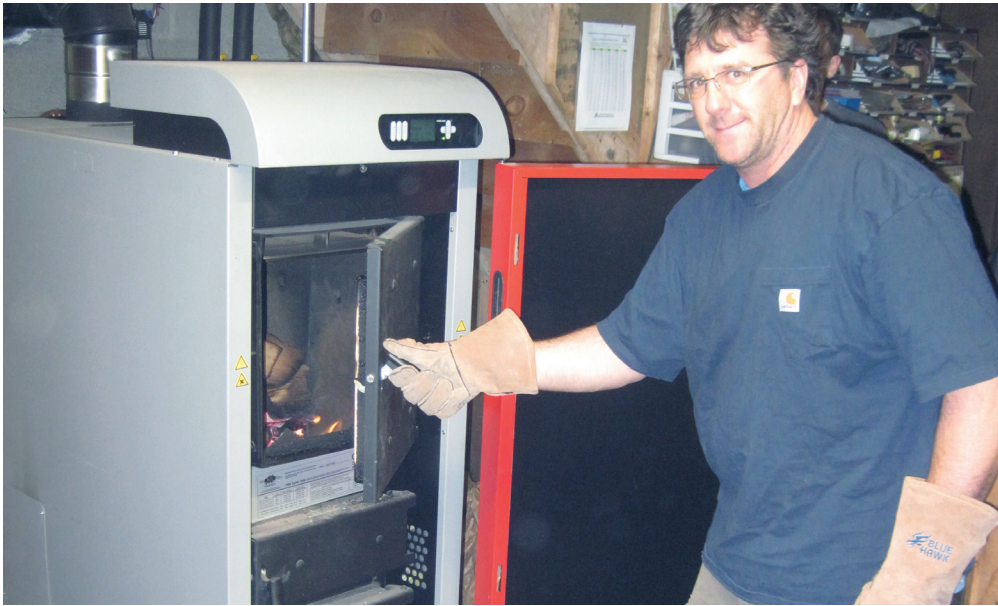
Mark Bomba adds cordwood to his father's new advanced cordwood boiler. Photo credit: NYSERDA
