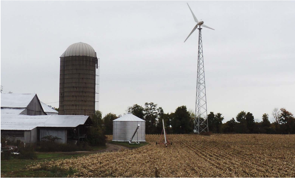
Endurance wind turbine at Ledge Farms. Credit: NYSERDA
