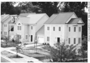
An example of a photovoltaic power system: The townhouse on the right, located in Bowie, Maryland, has a building-integrated photovoltaic (PV) standing-seam roof; the PV modules look and perform like the standard metal roofing on the other units, and they produce clean electric power.
