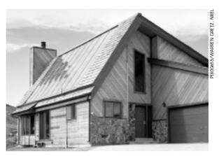
An example of a solar thermal system: The collectors for a flat-plate, solar thermal water heating system have been installed on the roof of this house in Golden, Colorado.
