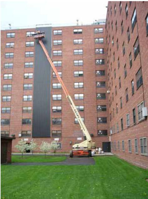
**Figure 5: Completing the cladding (Day 5)**
