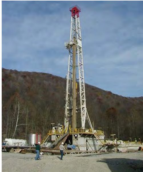
Active Well Drilling – Source: All Consulting
