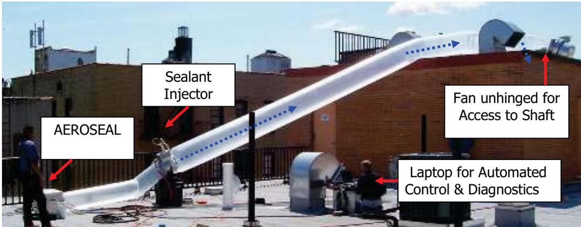
**Figure 1. AEROSEAL installation set-up on roof a demonstration building.**
