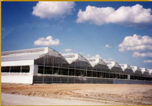
Proper heating and cooling are challenging design considerations. The major problem with heating is the energy cost. Facility design needs to consider maximization of heating efficiency while allowing for adequate ventilation. Ventilation (cooling) is a technical problem in many climates.
