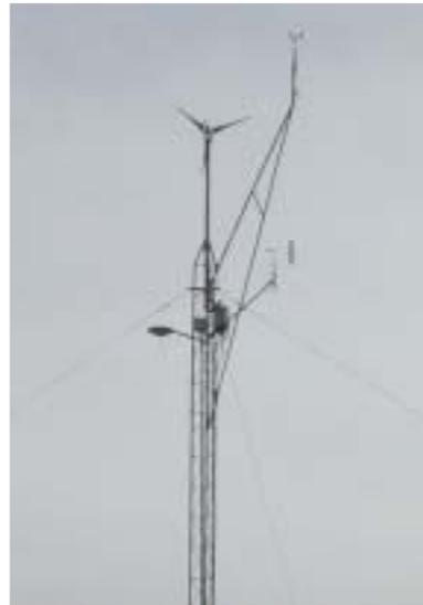
Southwest Windpower, Inc., of Flagstaff, Arizona, ([www.windenergy.com](http://www.windenergy.com)) produces the *AIR 403* (shown above), a three-blade upwind turbine with a manufacturer's rated power of 400 watts at 12.5 m/s. The DC output of the turbine was connected to a DC bus that was also connected to a battery bank and an Enermaxer. This device maintained the DC bus voltage at a constant 13.2 volts to prevent the turbine from shutting
