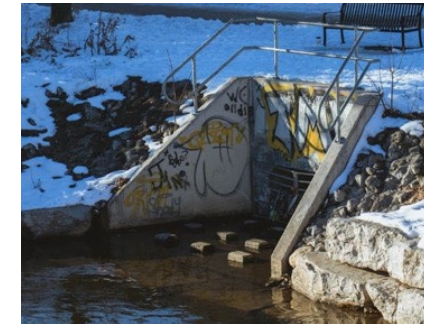
Storm and sewer
